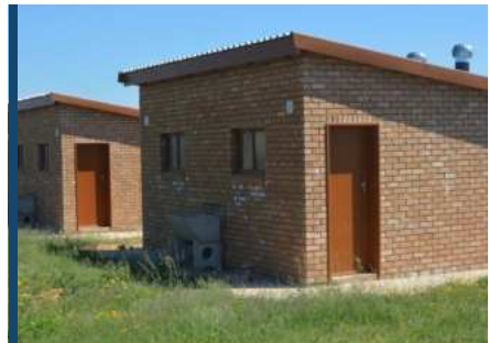
The newly built toilets at Klass Mothapo Secondary School, Limpopo.
