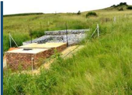
The spring water development project in Piet Reef, Mpumalanga.
